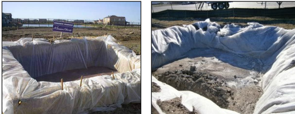
Plate 3-1 Typical concrete chute wash out areas
