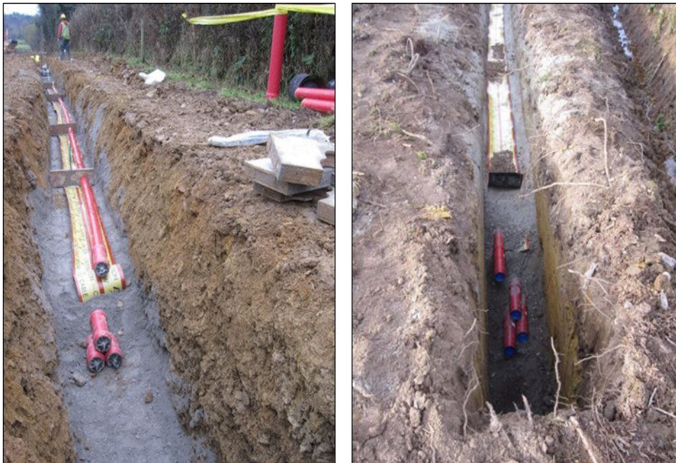
Plate 2-1 Cable Trench View
